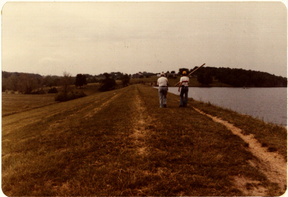
PHOTO NO. 7 - CREST TAKEN FROM LEFT END
