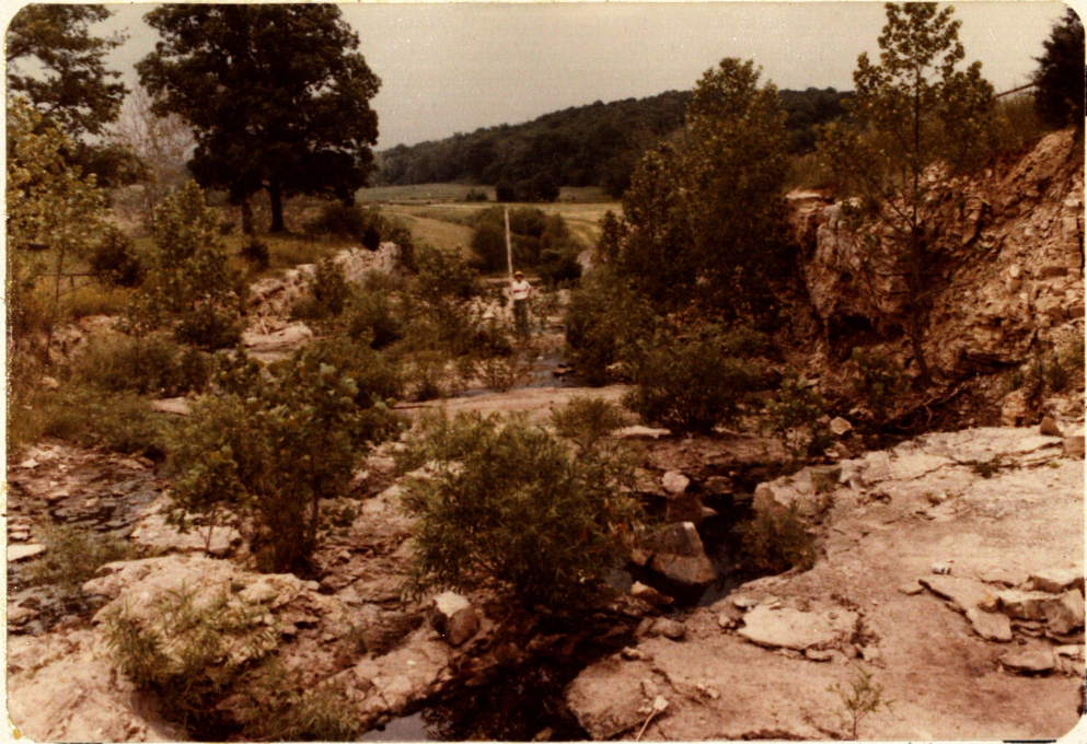
PHOTO NO. 12 - TAKEN FROM CONCRETE SILL LOOKING DOWNSTREAM IN PRINCIPAL SPILLWAY
