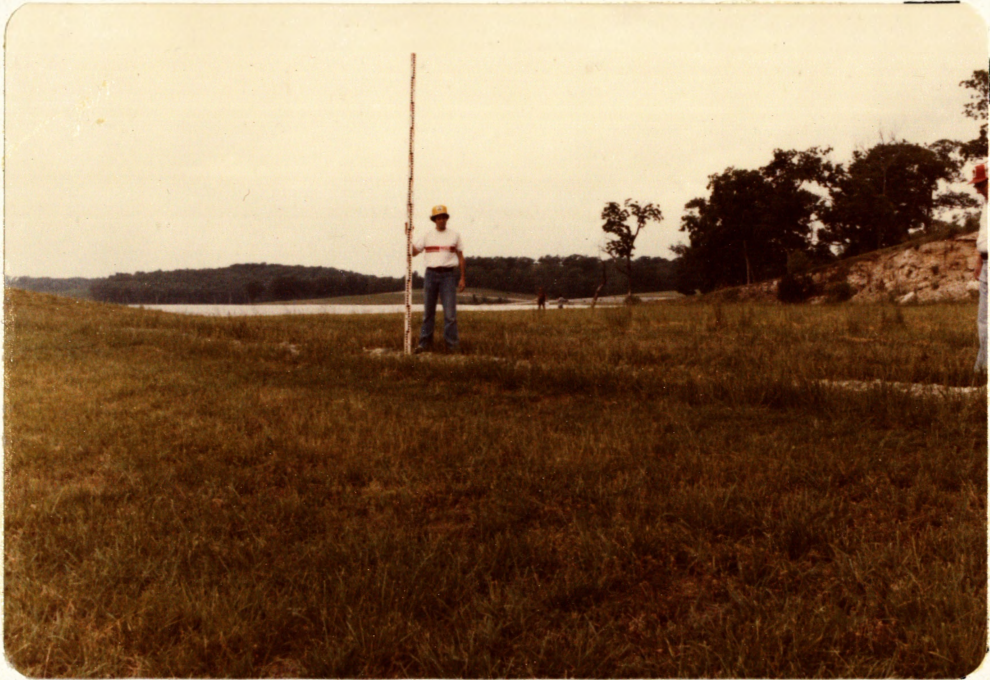
PHOTO NO. 4 - LOOKING UPSTREAM IN EMERGENCY SPILLWAY
