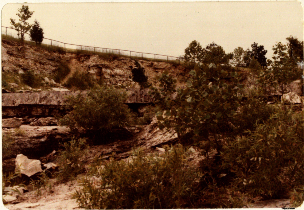
PHOTO NO. 13 - PRINCIPAL SPILLWAY CONCRETE SILL. PHOTO TAKEN FROM DOWNSTREAM
