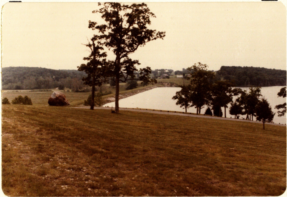
PHOTO NO. 2 - OVERVIEW TAKEN FROM UPSTREAM LEFT ABUTMENT
