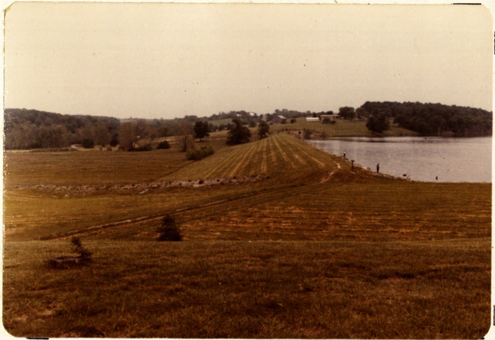
PHOTO NO. 16 - CREST AND DOWNSTREAM SLOPE FROM LEFT ABUTMENT
