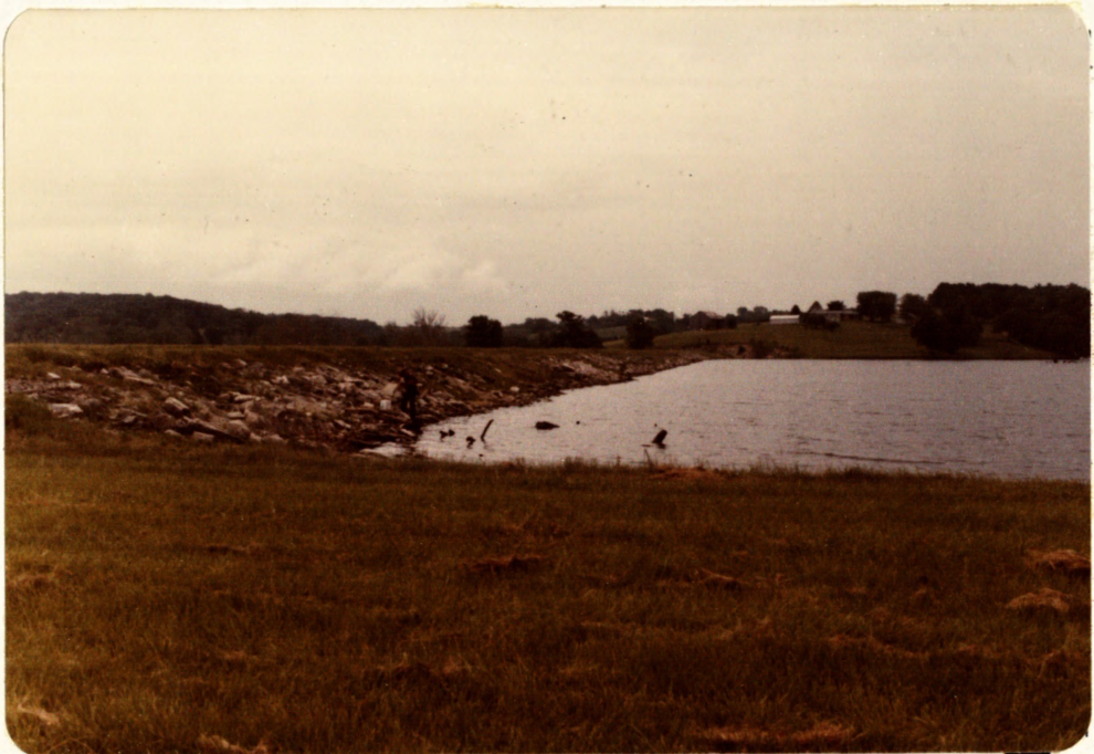
PHOTO NO. 5 - UPSTREAM FACE TAKEN FROM LEFT IN EMERGENCY SPILLWAY
