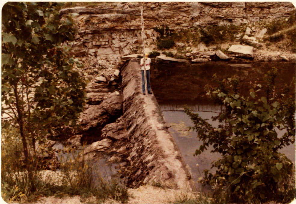
PHOTO NO. 11 - PRINCIPAL SPILLWAY CONCRETE SILL TAKEN FROM TOP OF DAM
