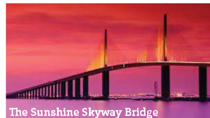
The Sunshine Skyway Bridge
