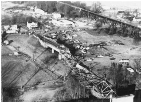
The Ohio River Silver Bridge After Collapse on December 15, 1967 [2]
