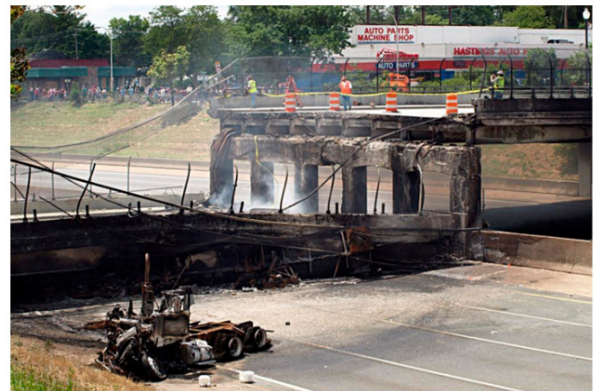
Fig.2 Fire-induced girder collapse Hazel Park overpass in Michigan [3]
