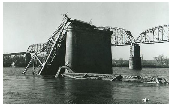
Deadliest Bridge Disaster in US History Caused by 2.5 Millimeter Deep Crack [7]
