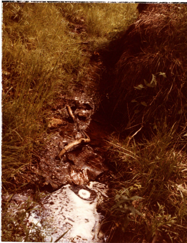
6. Total seepage and overland drainage below toe of dam. Looking east.
