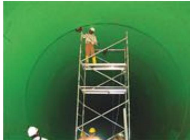
Measure thickness of concrete layers
