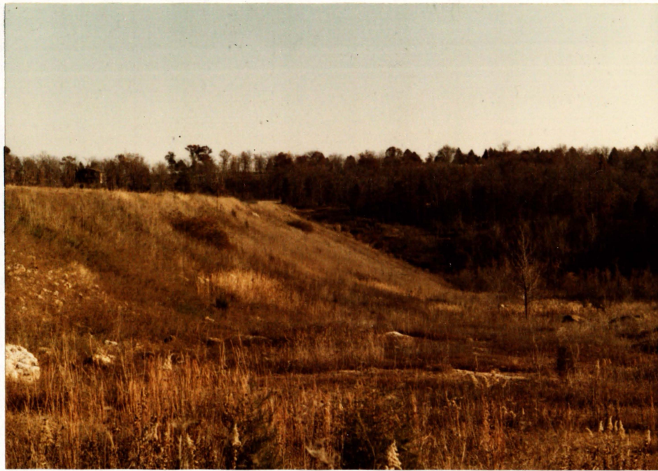
5. Downstream slope of dam showing grass and weed cover. Looking southeast.
