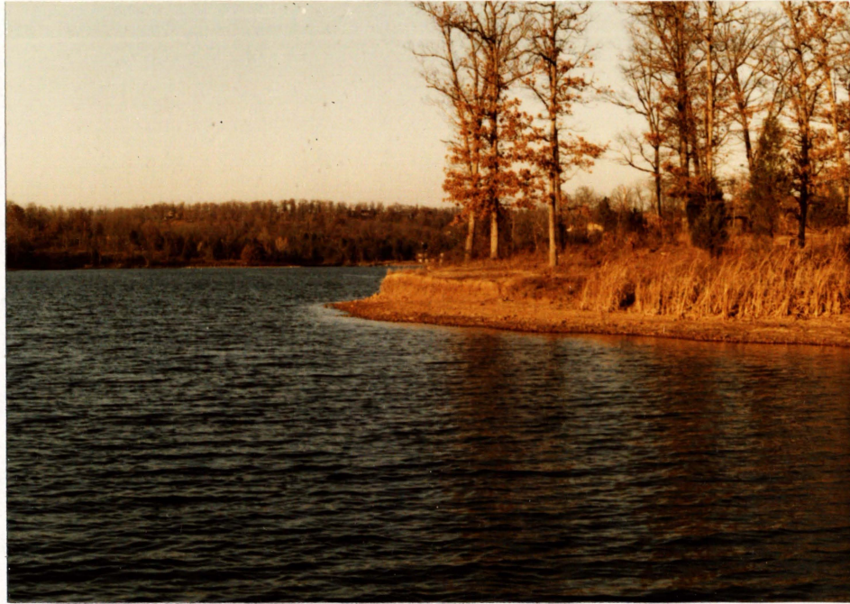
11. Wave-notched shoreline. Eroded to shallow bedrock, approximately 3 ft. Looking north from left abutment.
