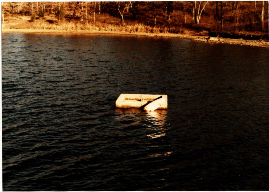
9. Top of concrete inlet tower for pipe outlet facility near left (south) abutment. Looking northeast from crest of dam.
