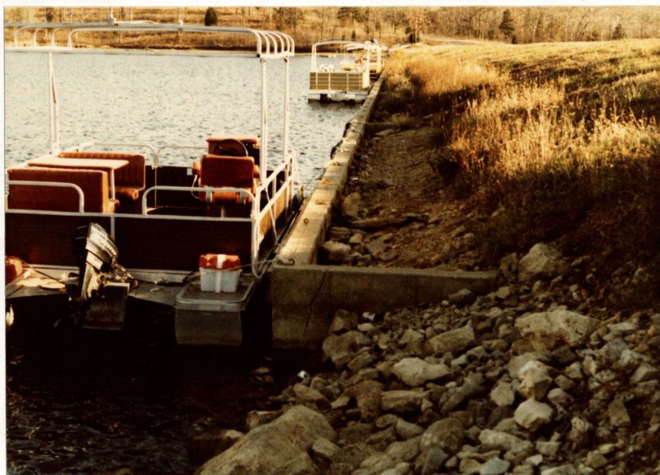
4. Concrete mooring wall along center third of dam. Looking southeast.
