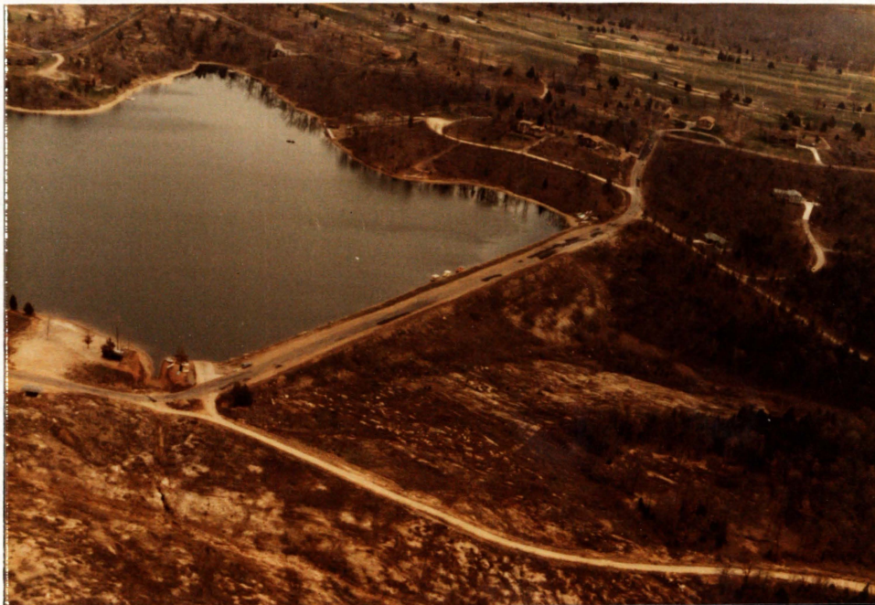
12. Discharge channel area in lower left of photo. Channel flows on exposed bedrock for most of its length. Note that discharge is routed well away from toe of embankment. Looking east.
