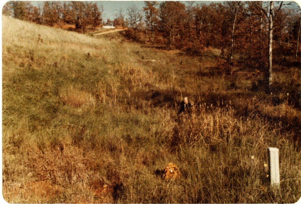
PHOTO NO. 14 - CATTAIL AREA AT TOE OF DAM (STA. 3+00 to 3+50)
