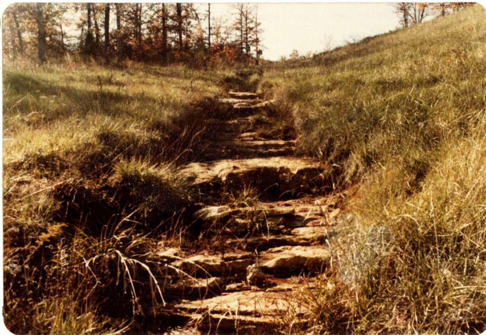
PHOTO NO. 13 - LOOKING UP SPILLWAY EXIT CHANNEL IN RIGHT ABUTMENT TROUGH
