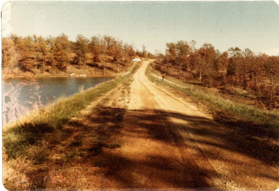
PHOTO NO. 12 - DAM CREST FROM RIGHT END
