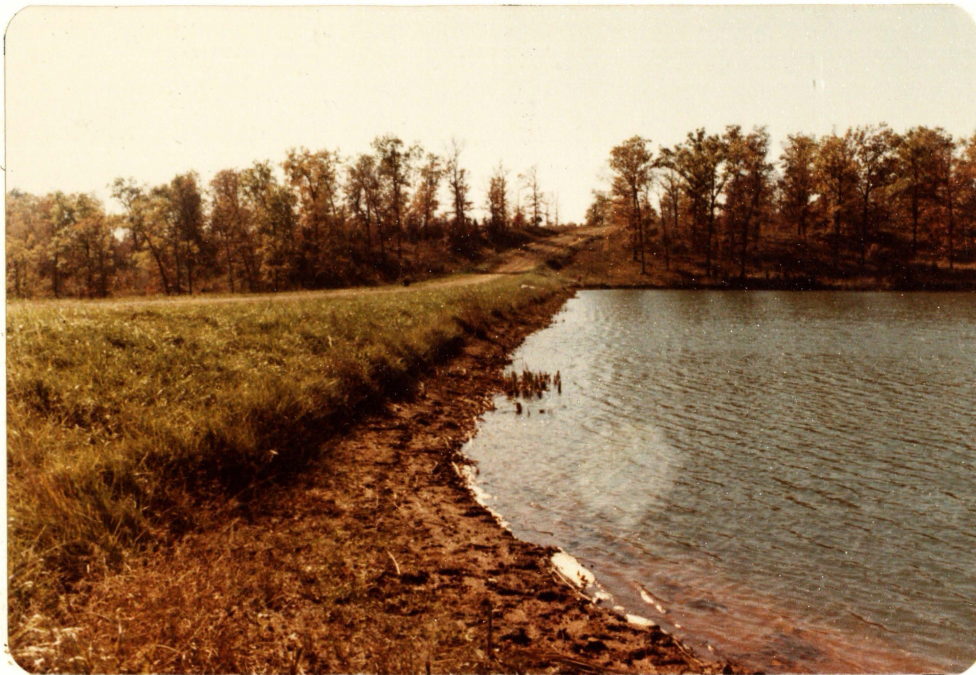
PHOTO NO. 5 - UPSTREAM SLOPE FROM THE LEFT END
