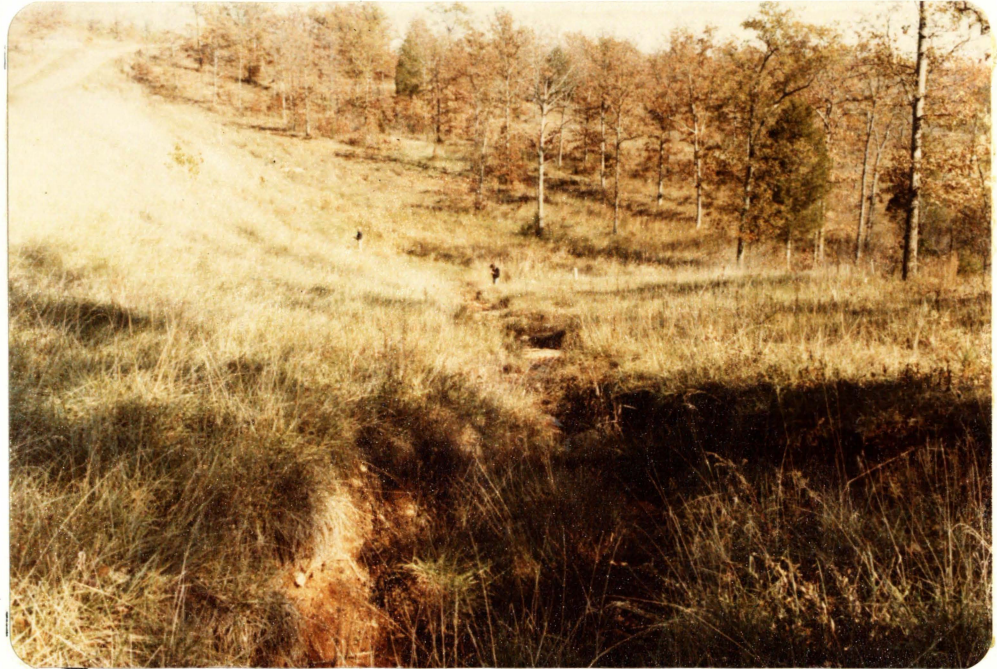
PHOTO NO. 10 - VIEW LOOKING DOWN THE SPILLWAY EXIT CHANNEL (RIGHT TROUGH)
