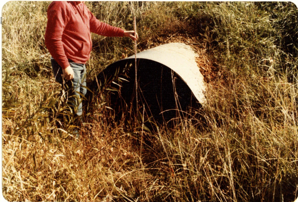
PHOTO NO. 11- INLET TO THE PRINCIPAL SPILLWAY PIPE
