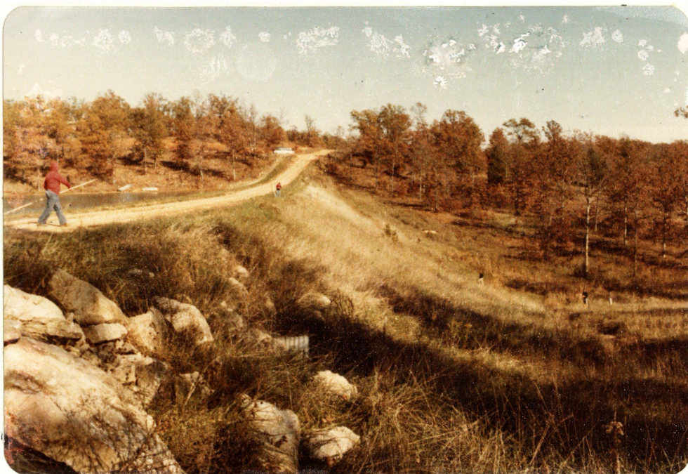
PHOTO NO. 8 - DOWNSTREAM SLOPE TAKEN FROM RIGHT END
