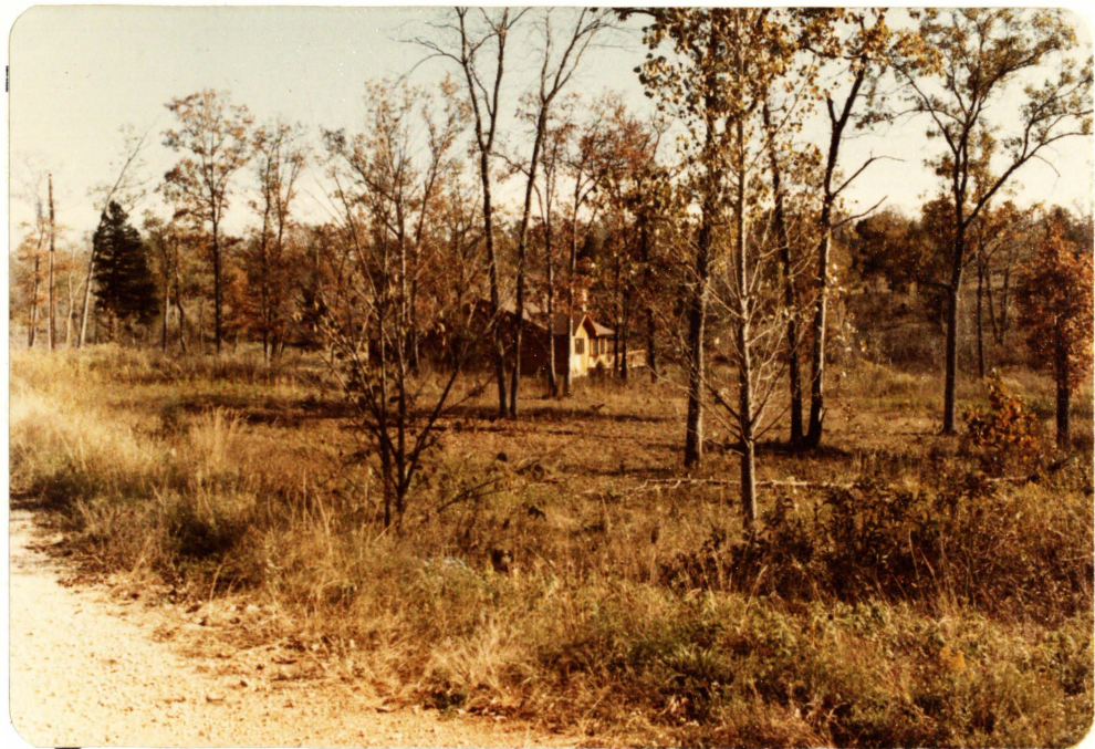
PHOTO NO. 19 - ANOTHER DOWNSTREAM HAZARD AT UPSTREAM END OF LOWER LAKE
