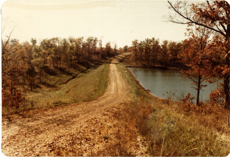
PHOTO NO. 4 - CREST FROM THE LEFT END
