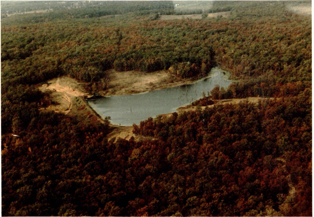
AERIAL VIEW OF LAKE AND DAM
