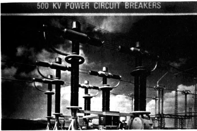
Figure 10. 500 kV Air Blast Circuit Breaker
