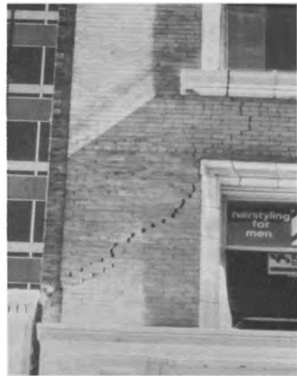
Fig. 17 Pounding Damage
