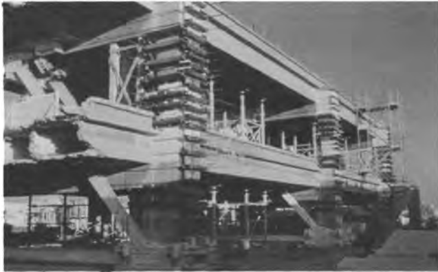
Fig. 26 Cypress Street Test Structure
