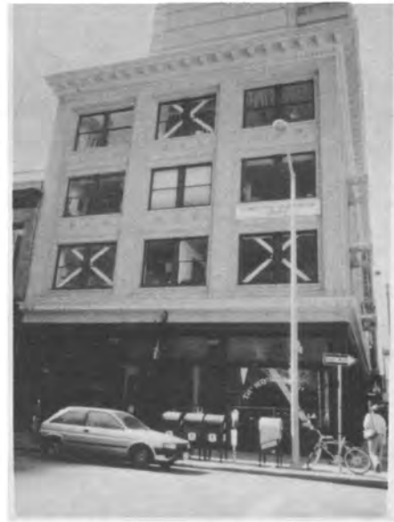
Fig. 15 Retrofit URM Building with Steel Braces
