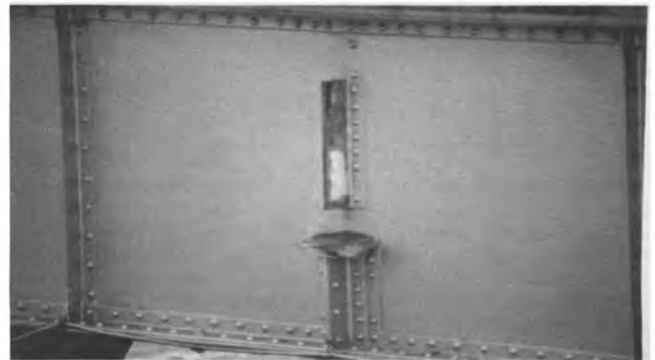
Fig. 19 Detail of Seat Connection on Bay Bridge
