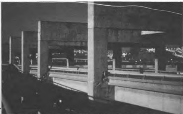
Fig. 24 Damage to Southern Freeway
