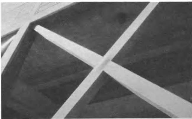
Fig. 12 Buckled Brace Intersection
