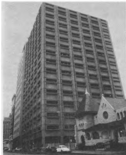
Fig. 10 Lightweight Concrete Shear Walls Failed at Base of Building
