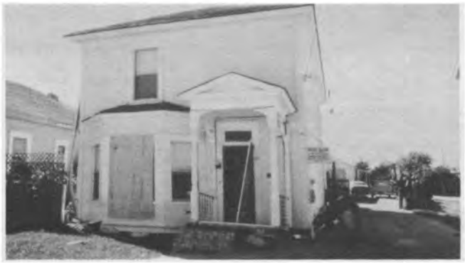
Fig. 4 Collapse of Home on "Pony" Walls
