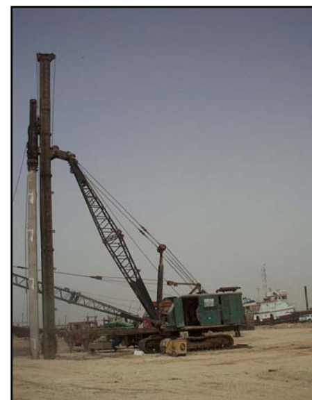
Fig. 3. Pile driving start
