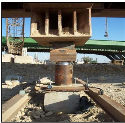
Fig. 4. Static loading test on pile
