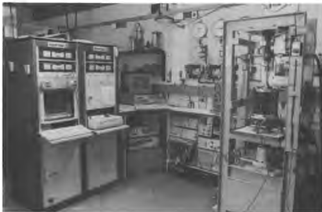
Fig. 2 Digital Control System
