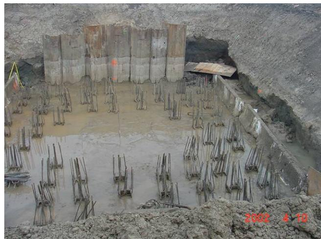
Fig. 7. Steel (H) piles after driving and retapping
