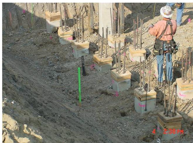
Fig. 6. Reinforced concrete pile driving
