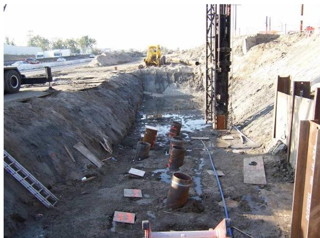
Fig. 5. Battered steel pipe piles ready for retapping
