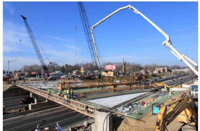
*Fig. 6 Bridge Deck Under Construction*
