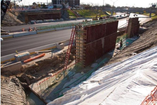
Fig. 3 West Abutment Footing and Wall
