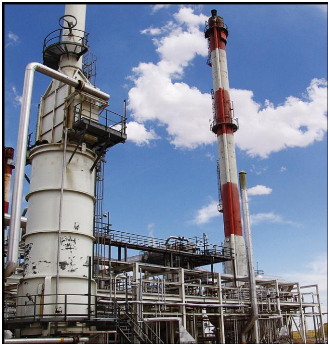
Fig. 1. Steel stack view
