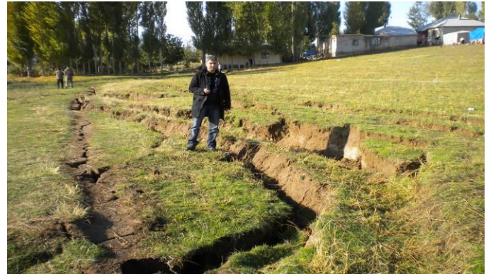
Fig. 4. Lateral spreading cracks in Celebibagi village (Ercis) affecting one-story masonry buildings at the background
