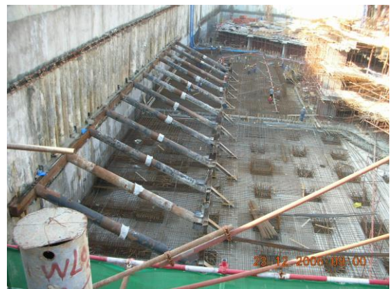
Plate 3. Installed Strutting System
