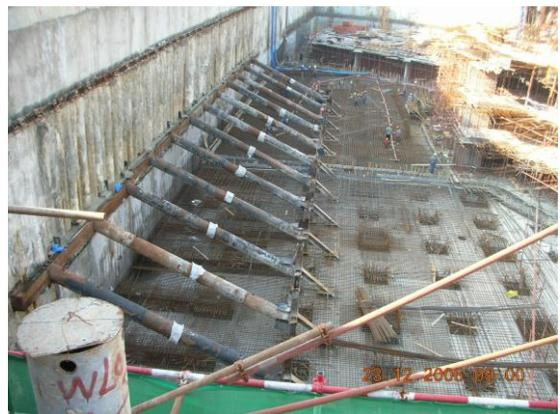
Plate 3. Installed Strutting System
