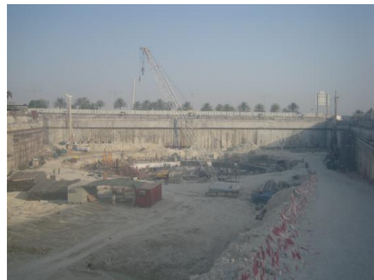
Plate 1. Excavation to Level of -12m
