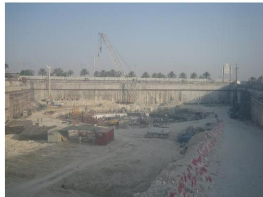
Plate 1. Excavation to Level of -12m
