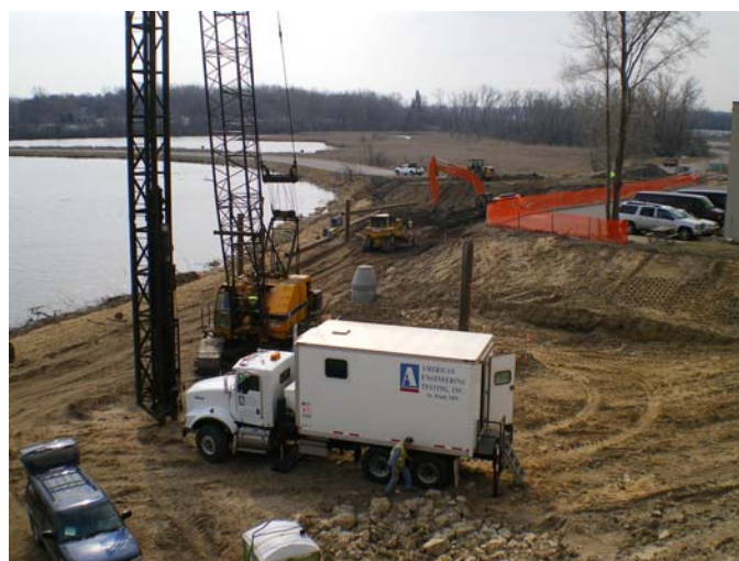
Fig. 1. SCPTu testing at the project site.
