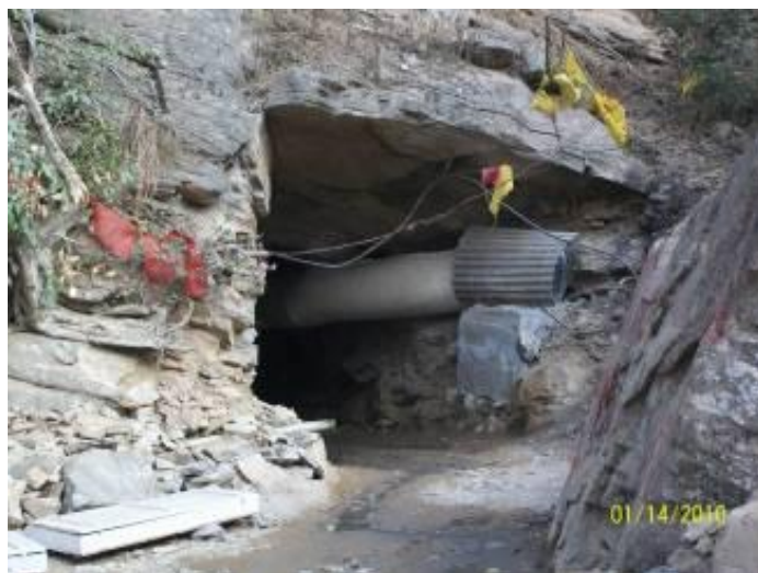
Fig. 3 Portal of the exploratory drift to desilting chamber, Punatsangchhu H.E. Project.
