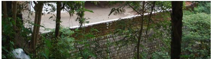
Fig. 10. Gravity masonry retaining wall
