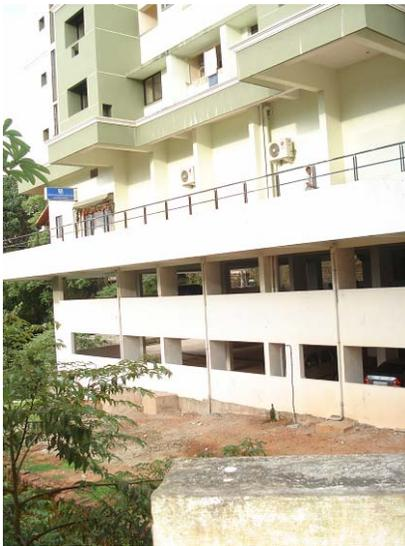
Fig. 6 Floor configurations suiting terrain
