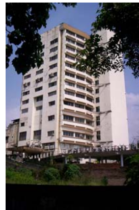
Fig. 1. Add on high speed lift shaft after restoration
