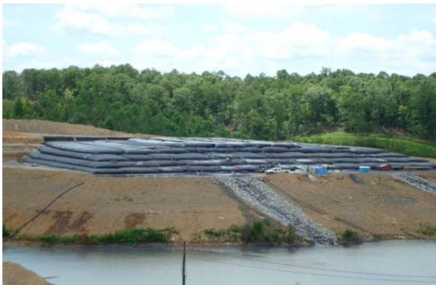
Fig 5. Sediment disposal using flat geotubes (Zhu et al., 2010).
