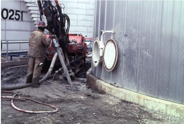
Fig. 11. Remedial grouting programme in progress
