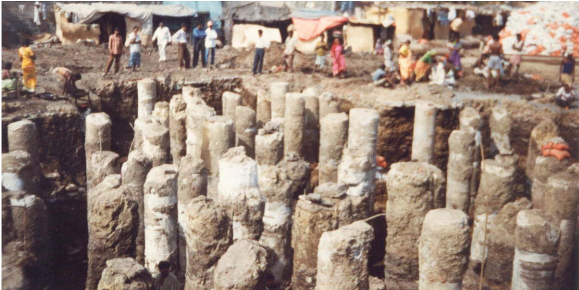
Piling on dumping ground at Worli, Mumbai.
