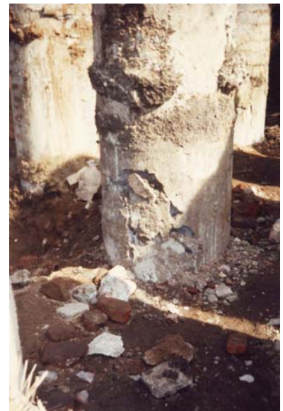
Site -Worli, Mumbai Piling on dumping ground
