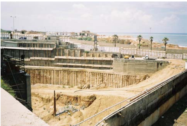
Photo 1 Excavation showing a shoring system in sand dune area
