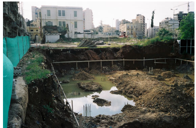
Photo 2 Excavation showing high water table in a red sandy area
