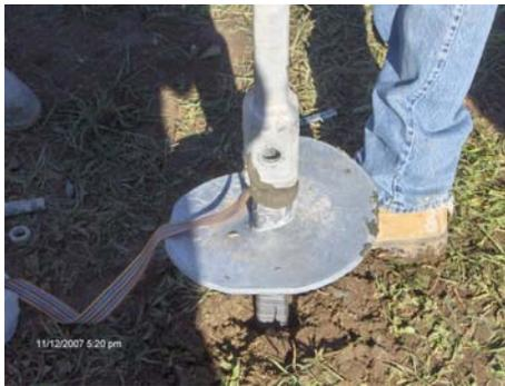
Fig.7. Typical preparation of lead section – extension connection
