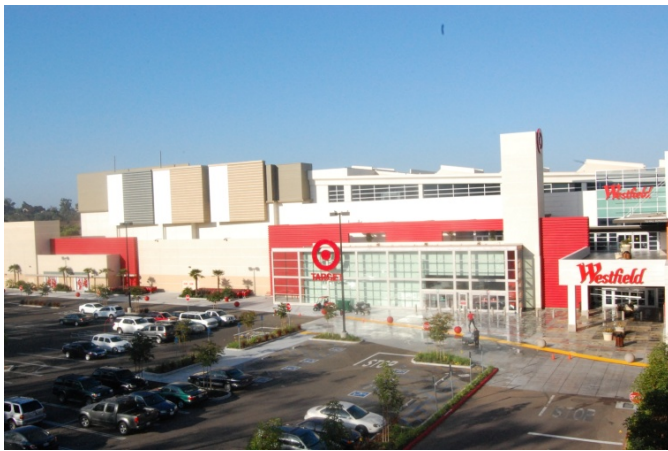
Fig 11. The constructed 230,000 ft 2 (21,367 m 2 ) addition at the Westfield Plaza Bonita shopping mall in San Diego, California, USA.
