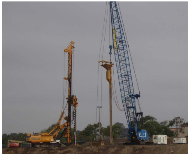
Fig 6. Equipment used for vibro stone column installation.
