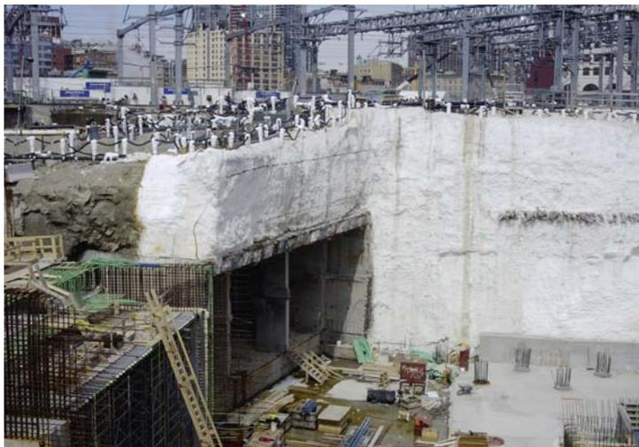
*Fig.10 Overall view of the frozen ground support walls and the completed base slab of the cut and cover tunnels.*
