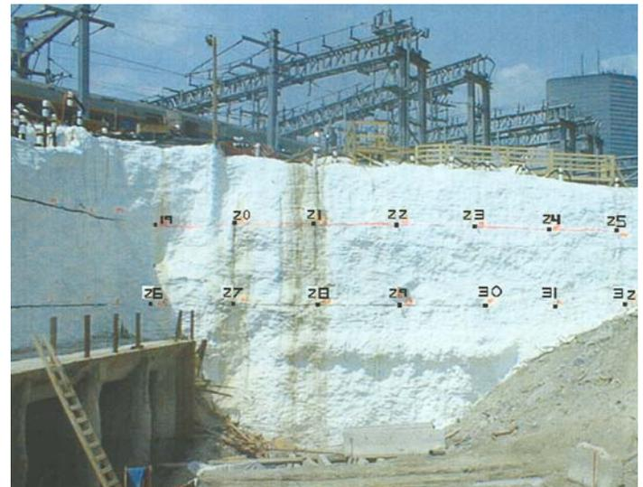
Fig.9 Overall view of the frozen ground support walls and Movement Monitoring Points on the Frozen ground Wall (also showing optical survey points on the exposed face of the frozen ground wall)
