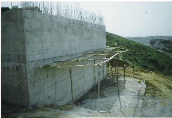
d) Construction near completion
