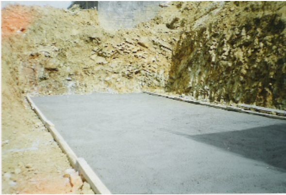
a) Foundation excavation
