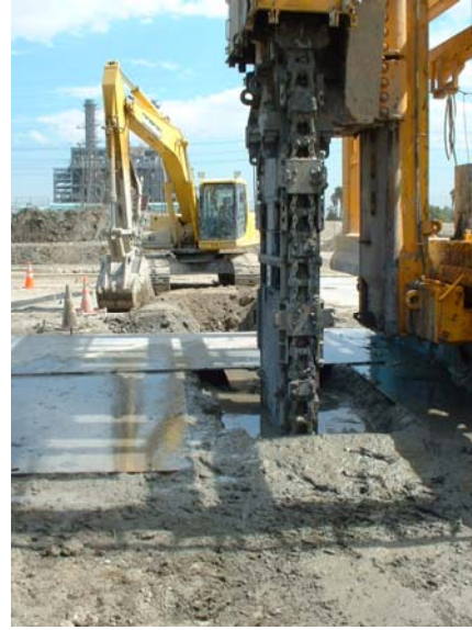
Fig. 1. Equipment for trench cutting and remixing with the TRD method at Alamitos Gap
