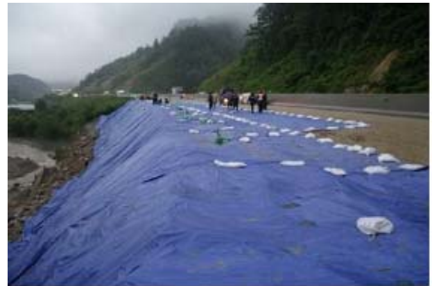
Pic.4 Vinyl mat was covered on the embankment
