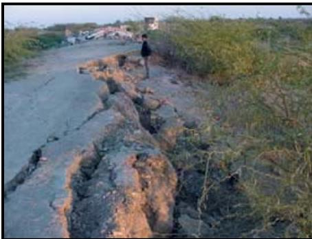
Figure 1d: Upstream slope failure of Fategarh Dam
