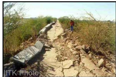
Figure 1a: Vertical and Crest settlement of Suvi Dam
