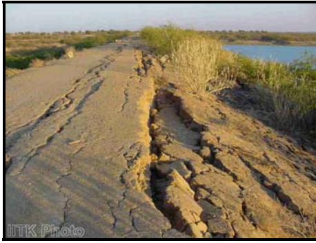
Figure 1b: Longitudinal cracks in the crest of Fategarh Dam
