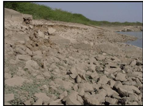
Figure 1h: Cracking and Slumping in the upstream face of Rudramatha Dam
