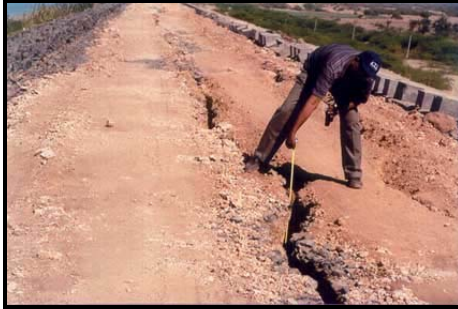
Figure 1b: Longitudinal cracks in the crest of Fategarh Dam
