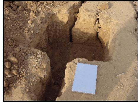
Figure 1f: Longitudinal cracks in the crest of Kaswati Dam
