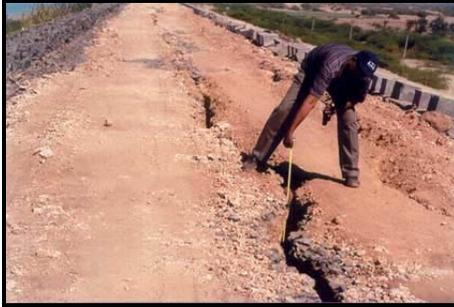
Figure 1c: Longitudinal cracks in the crest of Tappar Dam
