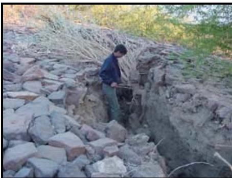
Figure 1e: Massive cracks in the upstream embankment near the toe of the Fatehgarh dam
