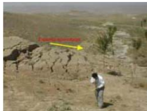
Figure 12. Slumping of the left bank of river at upstream side
