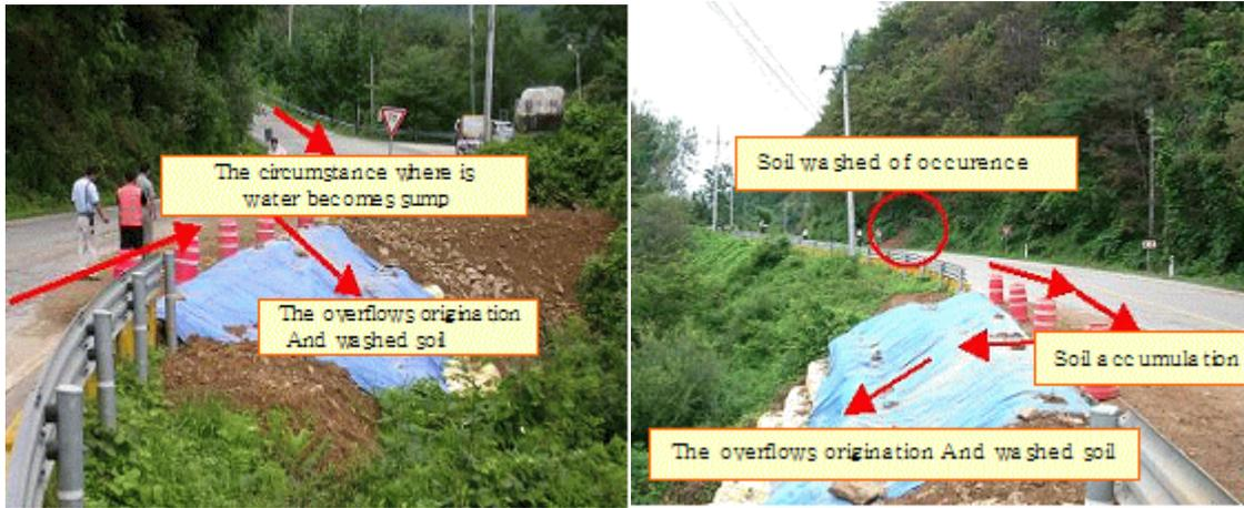
**Fig 10. The damage example due to washing of fill material**
