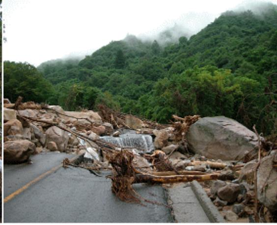
**Fig 18. Loss of road example**
