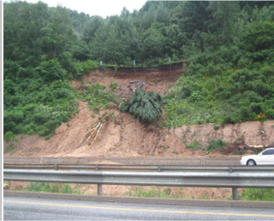
**Fig 8. Picture of arc type failure**
