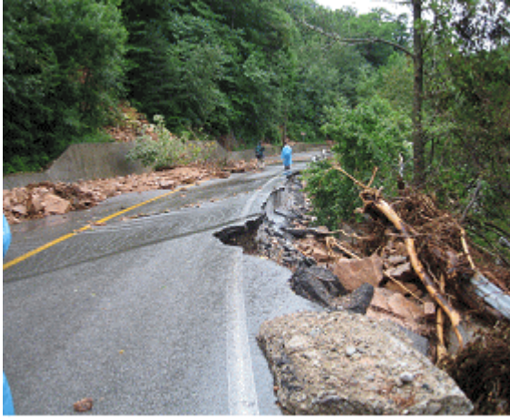
Fig 17. Loss of road by the boulder flow
