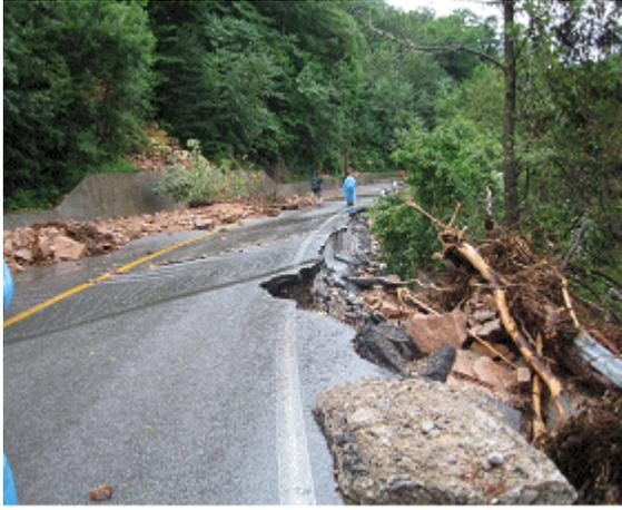
**Fig 17. Loss of road by the boulder flow**
