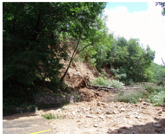
Fig 6. Picture of slope failure due to surface runoff
