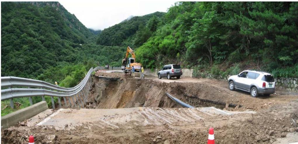
**Fig 9. The damage example by banking section**
