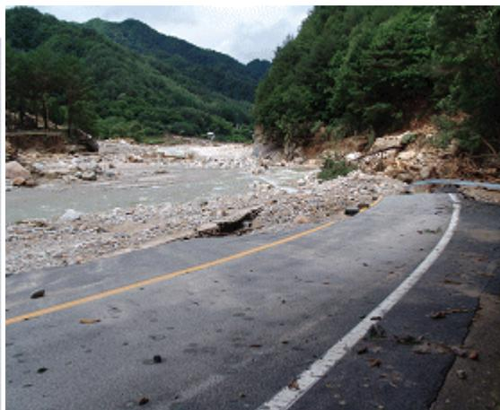
**Fig 12. Picture of failure due to water impact**
