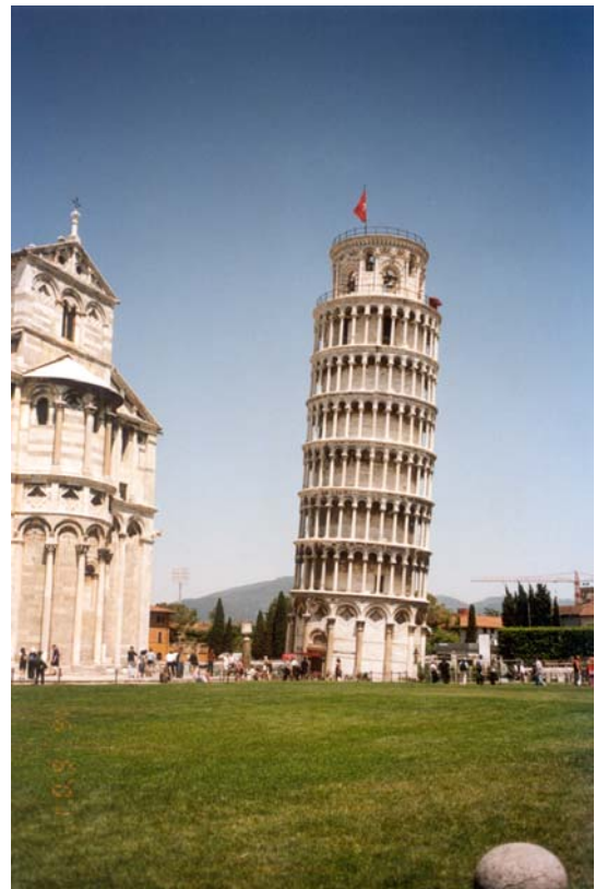
Fig. 1. The Leaning Tower of Pisa
