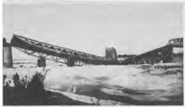
Figure 5. Overturning of Girders of a Railway Bridge During Bihar Earthquake of January 15, 1934.
