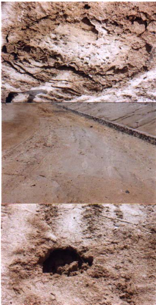
Fig. 7 Location from where the salt and water oozed out at salt factory at Bachau
