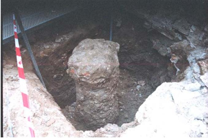
Fig. 6. Jet-grouting column.
