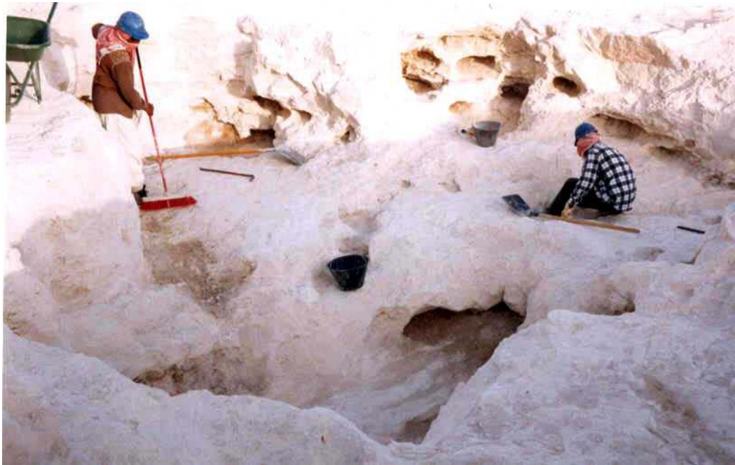
Plate: 3 Preparation being made for Treatment of Sinkhole at the Site
