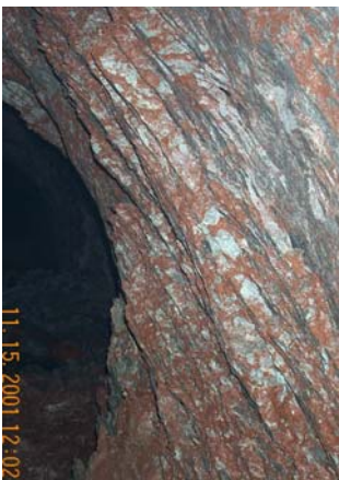
Fig. 4. Side wall scaling in 1751m cross-cut drift
