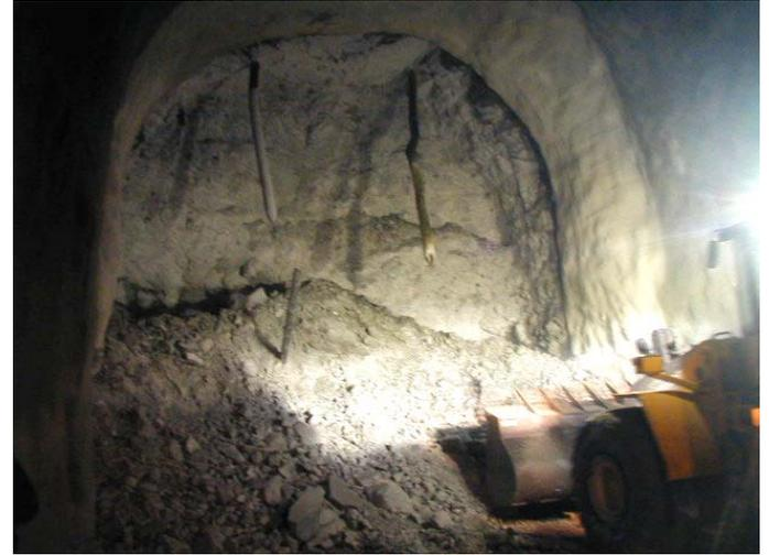
Fig. 9. Tunnel end after blasting. The cooling pipes for tunnel soil freezing were emptied before blasting.
