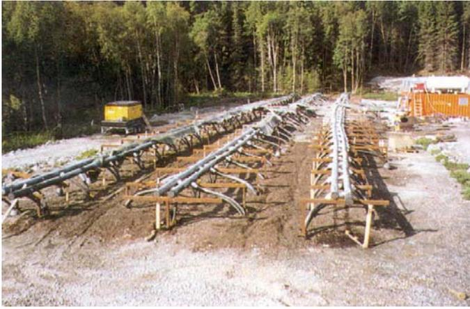
Fig. 7. Freezing installation on the ground surface, summer 2002.
