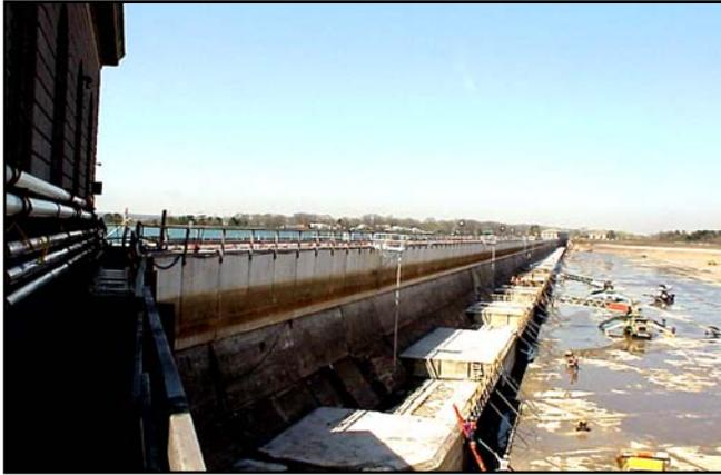
Fig.5. Buttress Construction in Checkerboard Fashion
