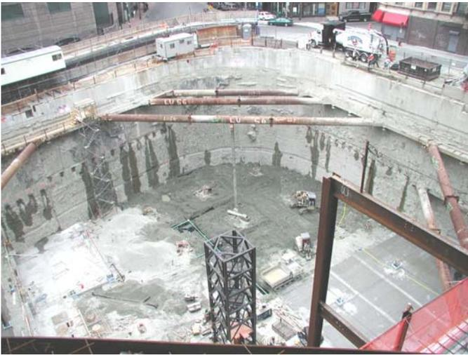
Fig. 9. The Arched Slurry Wall
