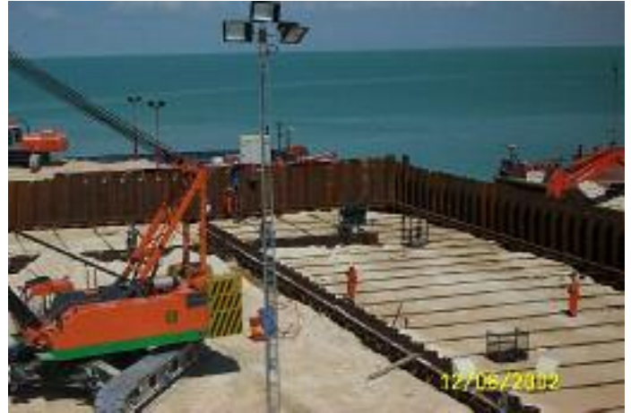
Figure 5. Installation of tie-rods
