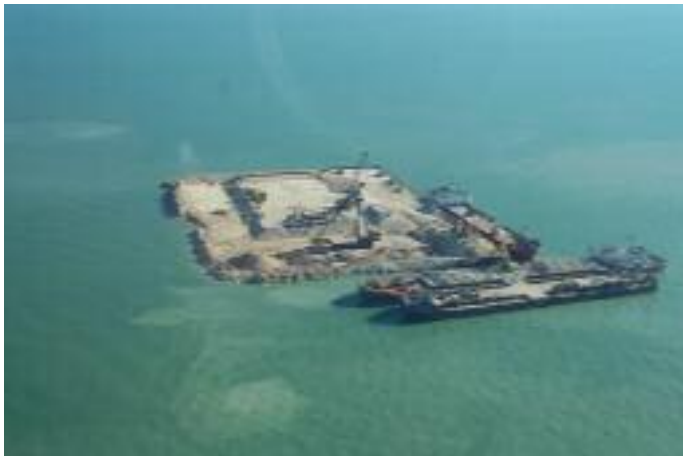
Figure 3. The panoramic view of the construction site
