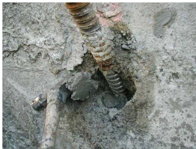
Fig. 10. Observed strut nail connection at existing wall.
