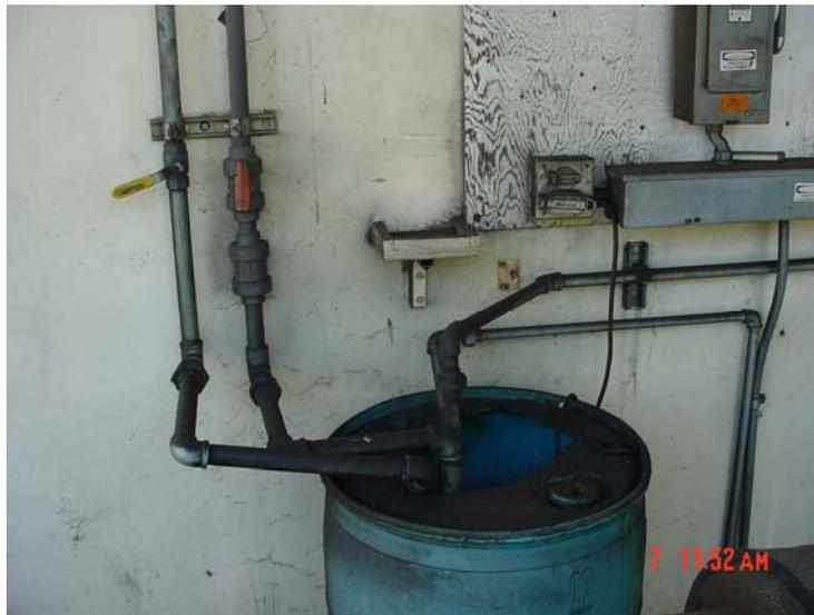
Figure 12 Drum for collecting condensation
