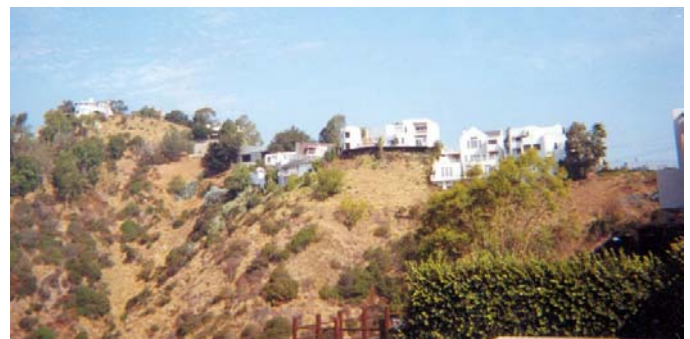
Fig. 2. Representative Hill-Side Site in the Northridge Earthquake Epicentral Area
