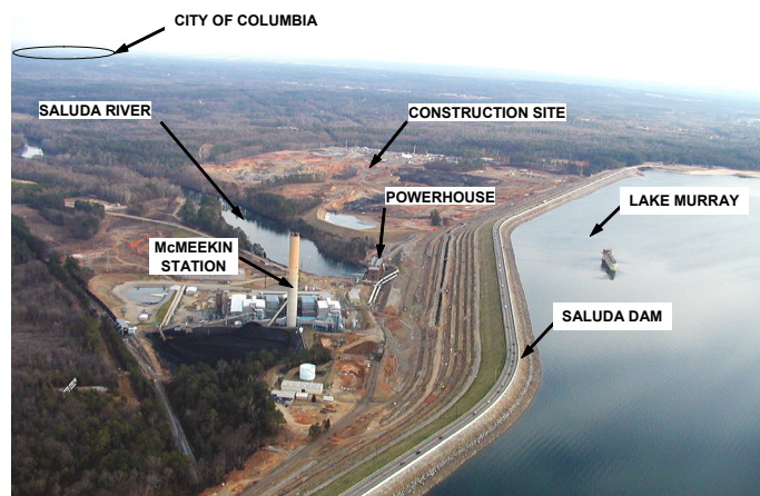
Fig.1. Saluda Dam and Project Overview.
