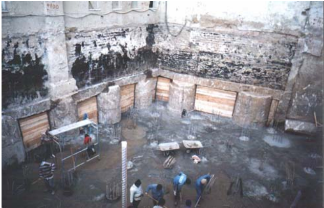
Fig. 6 Photo of the foundation of the existing building
