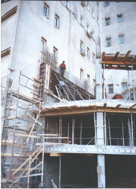
Fig. 10 Photo during the execution of the building extension
