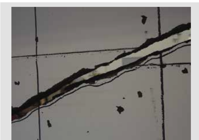
Figure 6. Shear crack in girder 2 from test 2.
