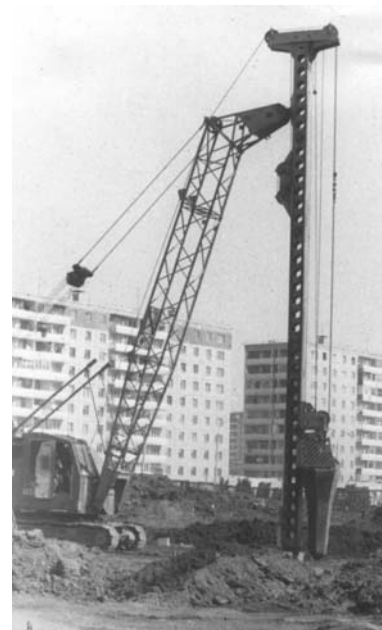
Fig. 2. General view of the unit and the tamper for the FTH construction on the site in the city Chelyabinsk
